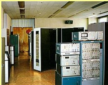
Multi-processor computing system PS-2000 (Lab. No. 31)
